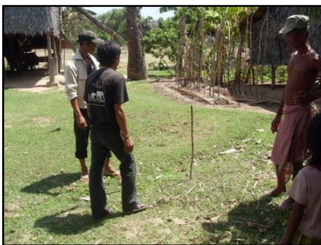
Left: Clean Water Project Manager, Somit shows the well contractor the new locations for drilling in Kork Por. Right: Drilling a new well in Kork Por.
