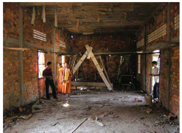
Construction of the future classroom.
